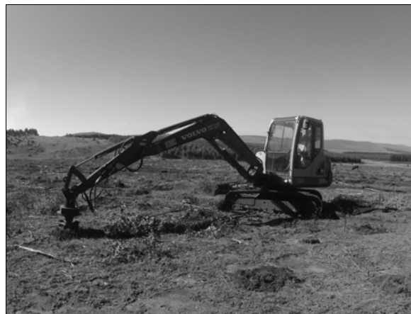
Figure 4. Modern mechanised pitting with mini excavator.
