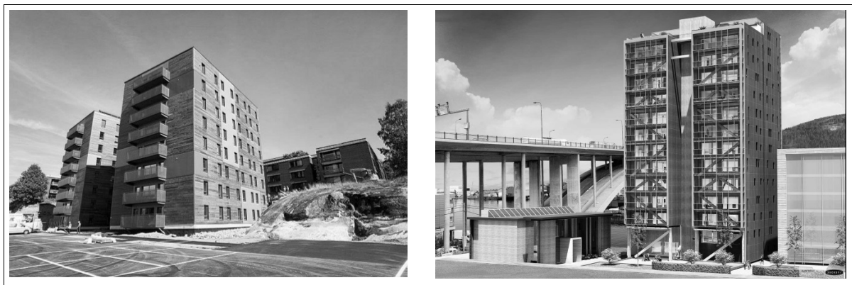
Figure 5. Left: 8-storey CLT-blocks for student-housing, Ås, Norway, finished 2013 (Photo: HåkonSparre, NMBU). Right: 14-storey combined CLT-modules and gluelam-frame, Bergen, Norway. Under construction 2014-2015 (Animation: 3Seksti/Artec/Sweco).
